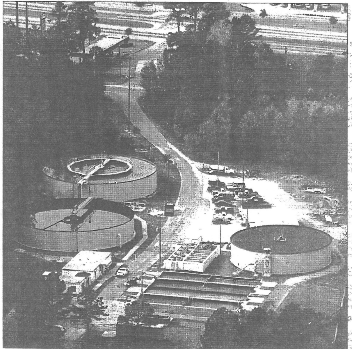
DAVE HAMBY/Staff Photographer The Lake Forest sewer plant in Daphne has been the focus of a continuing controversy in recent months over bay pollution.
